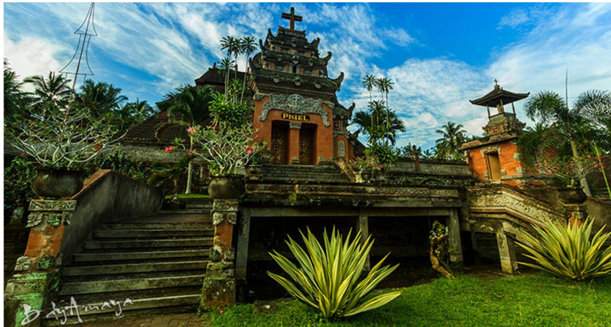
Picture 1 Balinese-style Church Building Source: Research Observation
